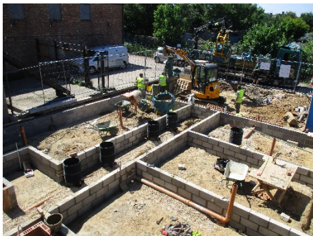
Photograph 11: Sub-structure blockwork underway
