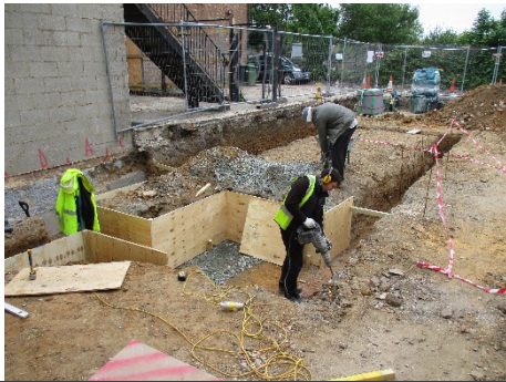
Photograph 9: Excavating foundations
