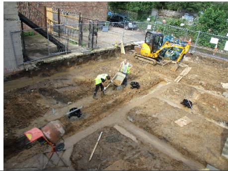
Photograph 10: Foundations poured
