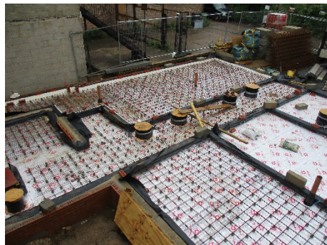
Photograph 12: DPM and insulation installed
